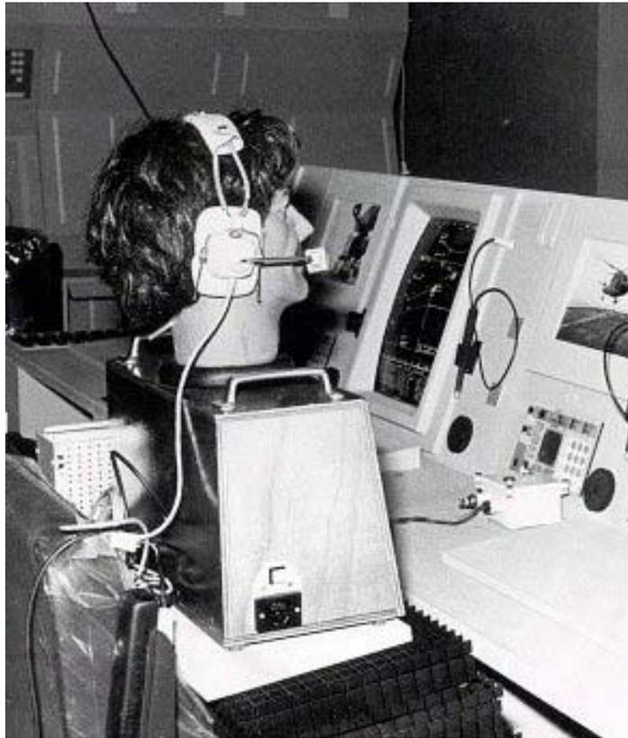
Figure 19. Artificial mouth used for the assessment of microphones.
